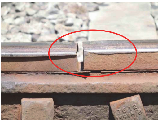
Figure 3.2.11 Deformation of Rail
