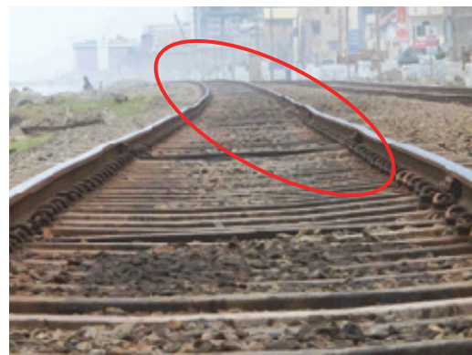
Figure 3.2.12 Irregularity of Alignment
