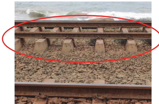
Figure 3.2.13 Exposed Sleepers
