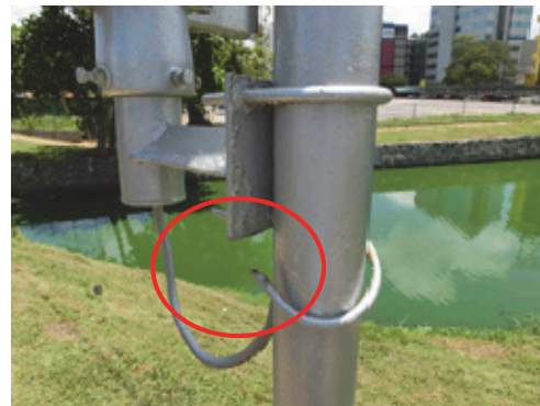
Figure 3.2.15 Exposed Terminal Box
